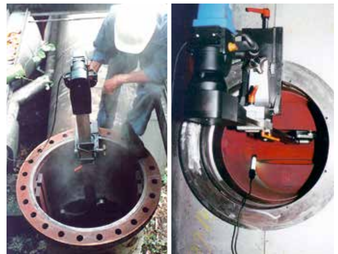
SHS 600 grinding on-site
