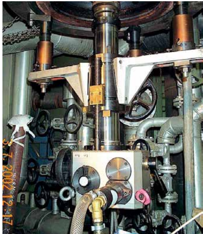
MD Application on site, overhead machining
